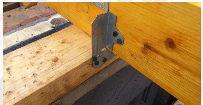
Method 2 – Fix truss to wall plate using truss clip
