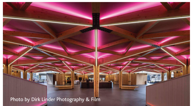
Structure showcasing the extensive use of Glulam and CLT
