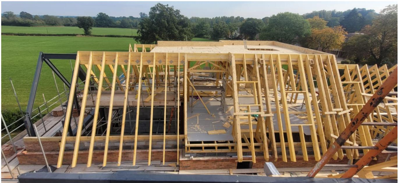
A steep 55° roof pitch was used to maximise head height in the attic and avoid dormer construction, helping the homes comply with local height restrictions. These homes feature vaulted ceilings above the hallways and master bedrooms, as well as multiple rooflights across both pitched and flat roof areas to enhance natural light.
